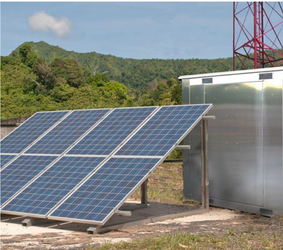
meeco sun2com installation
